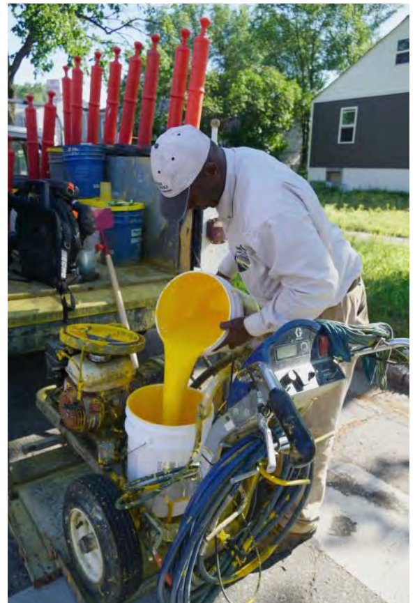
Bus Driver and Summer Painter Joseph Laurore pours paint at the Bismarck Early Childhood Center. The paint was used to create designated bus loading zones.
